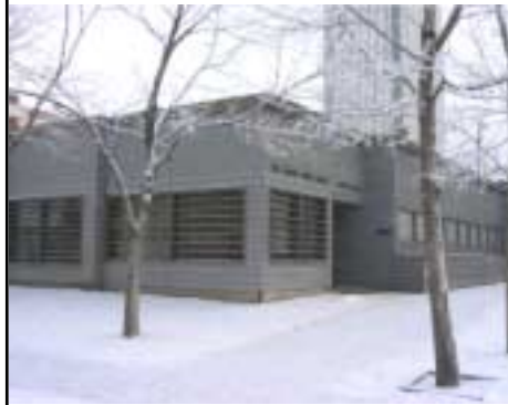
Spady Centre with capacity for 62 was overloaded for 6 years has added an addition costing $300,000 that added no extra mat space.
